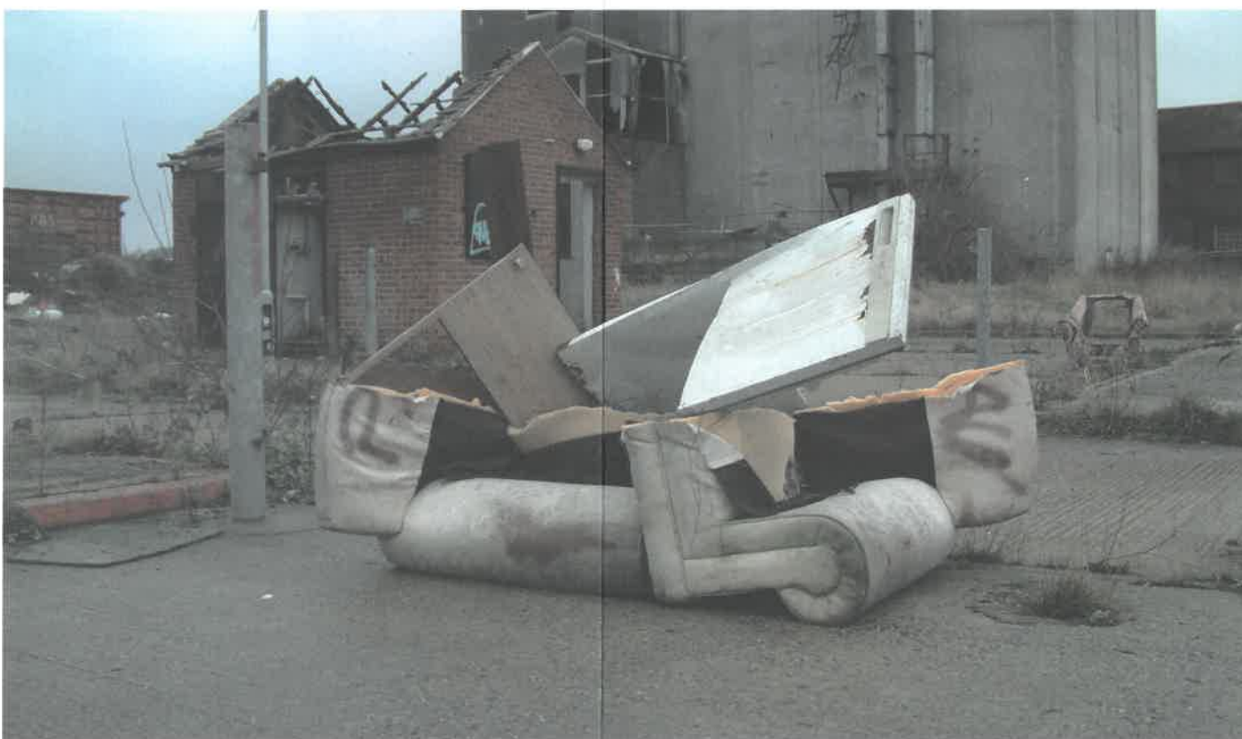
Hythe Demolition photograph 2003
